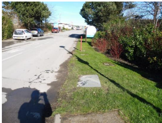
Main meter location
