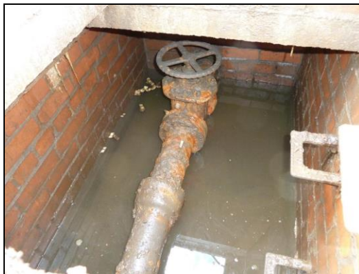
4" cast iron in chamber near gate house
