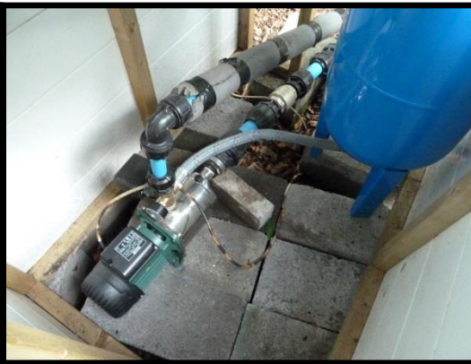
Picture 4 – Pump on outlet of large water storage tanks
