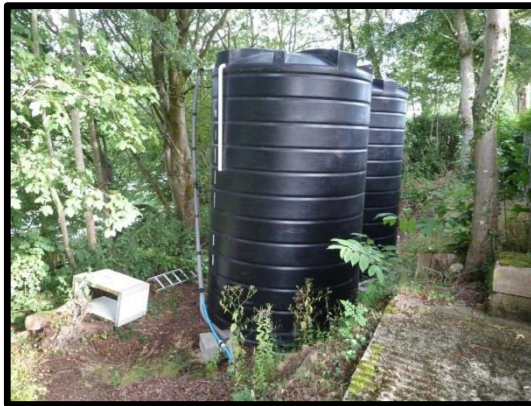
Picture 3 – Large water storage tanks & pump set
