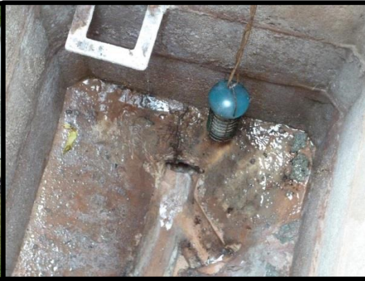
Picture 8 - Water breaking into drainage chamber
