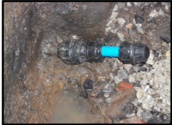
Picture 2 – The temporary repair on the supply pipe
