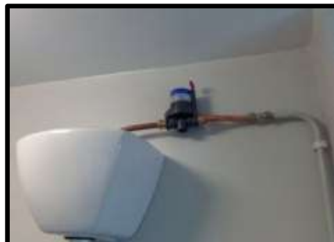
Picture 4 – The new cisterniser that has been fitted on site
