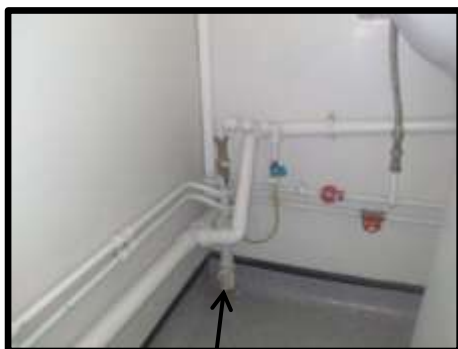
Picture 3 – The rising main enters the building in the toilet area
