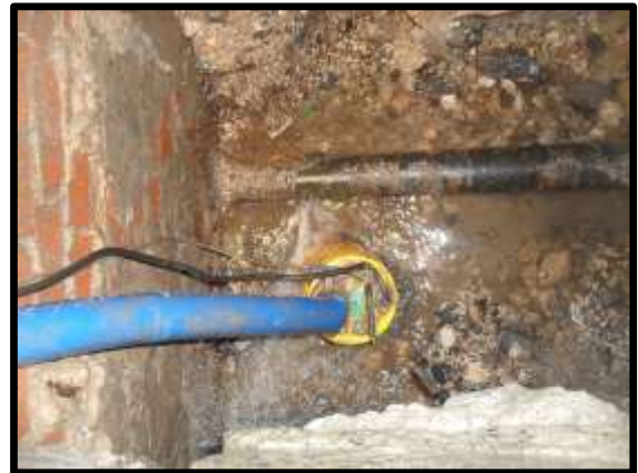
Picture 1 – The area of leakage in the fire hydrant pit
