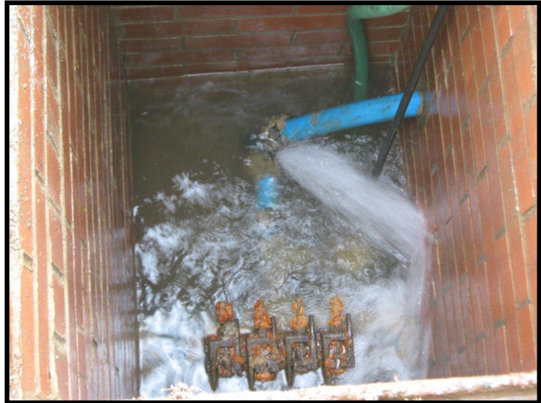
Pic 3 - Meter Chamber with leaking elbow joint
