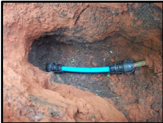
Pic 4 – The 32mm replacement plastic pipe that repaired the leak
