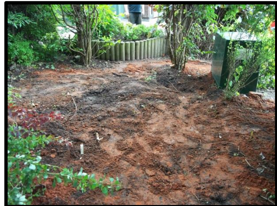
Pic 5 – The excavation area has been backfilled and fully re-instated
