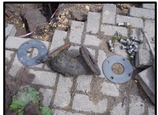
Picture 2 – T Joint Removed
