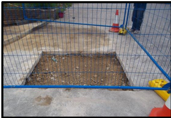
Picture 6 – Backfilled before Re-instatement
