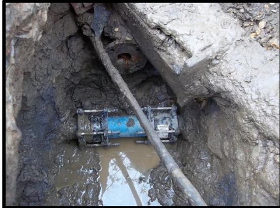
Picture 5 – Section of New Pipe
